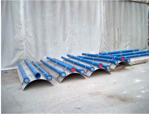
preassembled Rabtherm® - heat exchanger elements
