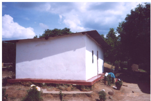
Fig.2 Cement sand plastered earth walls (Authors, 2004)
