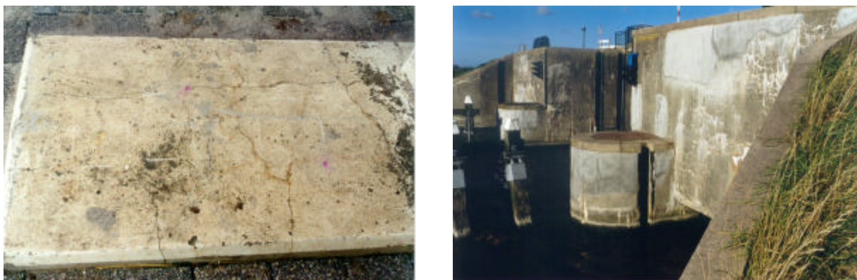
Figure 1: ASR-attack in the foundation of a viaduct (left) and a lock (right) in the Netherlands.
