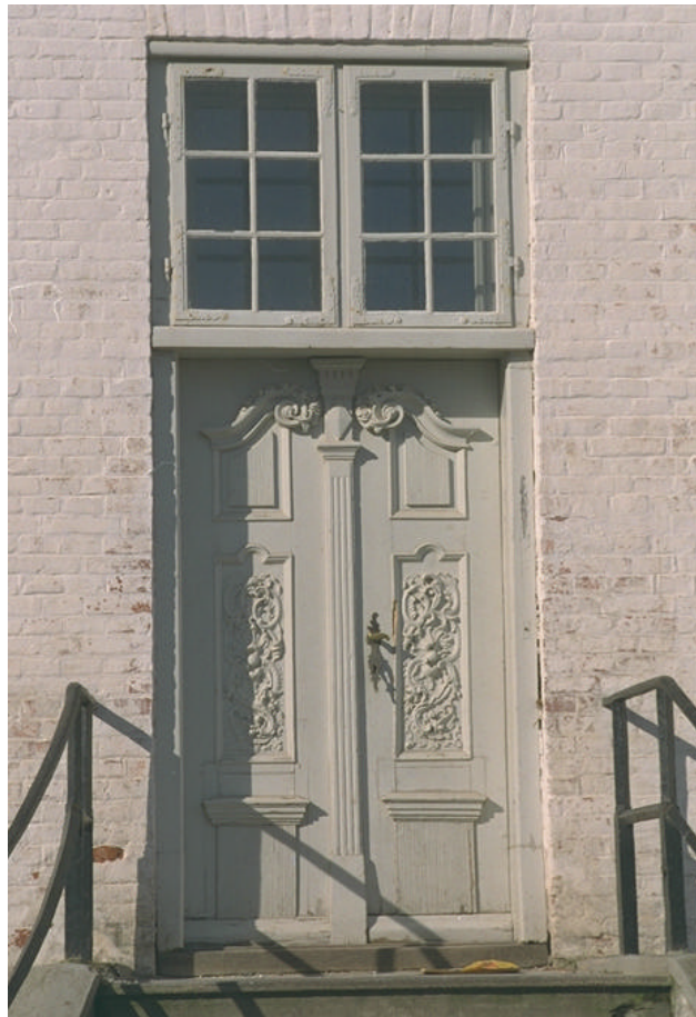
Figure 2. Linseed oil painted door with good performance after 8+ years. The wood quality is good and the workmanship of high quality.
