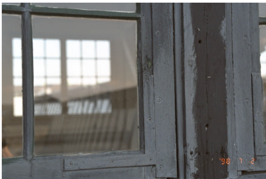
Figure 4. Repair of linseed oil painted window where the paint used for the repair differs significantly from the original due to a larger content of chalk filler.
