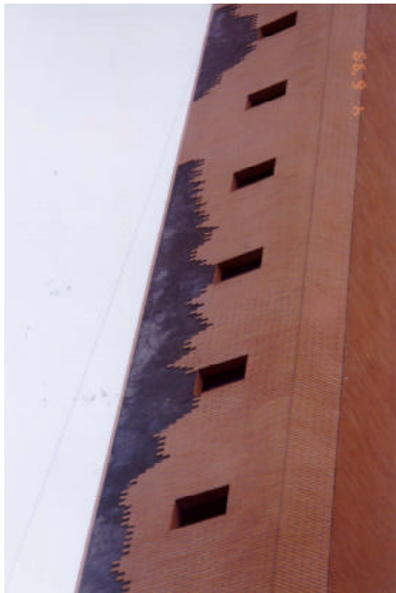
Figure 2: View of the façade affected by loose tiles
