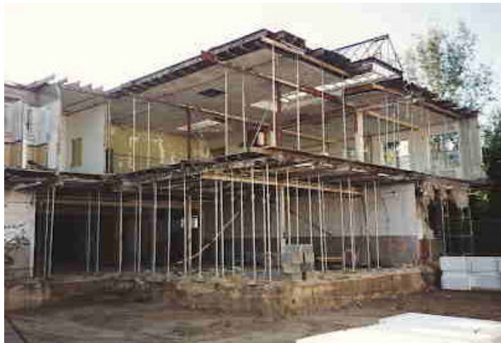
Fig. 1 A fully stripped building for re-use
