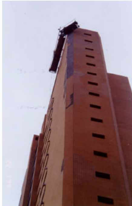
Figure 3: Evidence of lack of expansion joints on the right rear façade.
