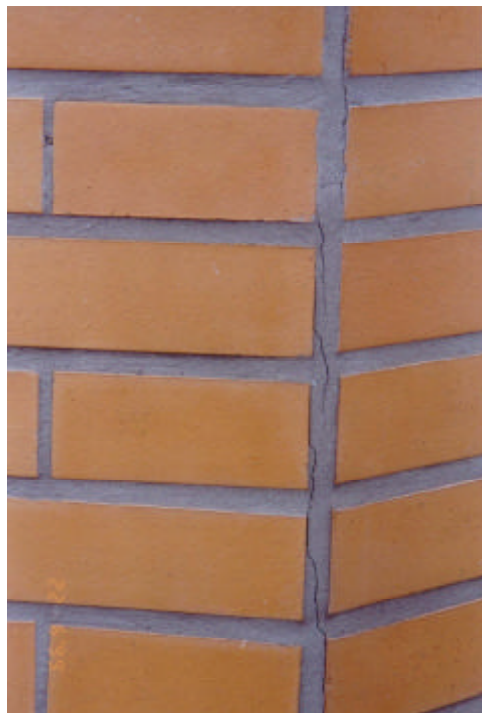
Figure 4: Evidence of cracks in the grouting between tiles.
