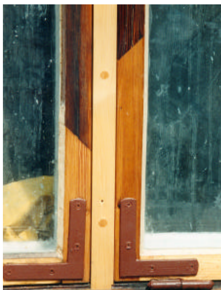
Figure 1. Mending of sashes in old wooden windows in order to preserve as much as possible of the original sashes.
