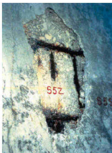
Figure 3. Vir Bridge - damage of the concrete pile
