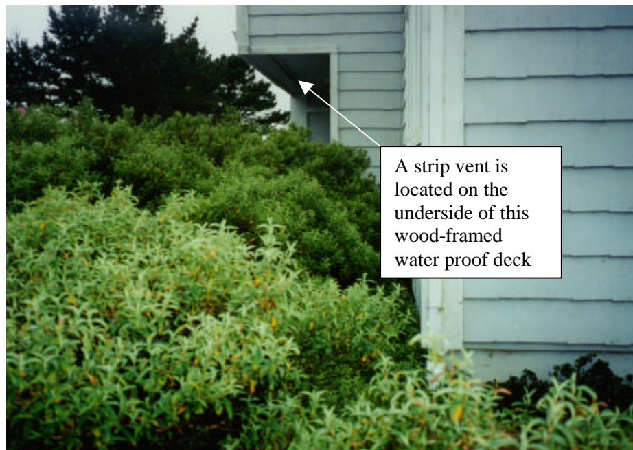
Figure 8. The strip vents commonly used in wood-framed waterproof decks are subject to the same flame and ember entry problems as crawlspace and attic vents. In this case, vegetation growing under the deck increases the potential danger to the structure.
