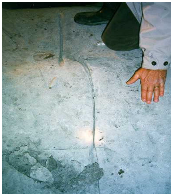
Figure 10: Back-side of the concrete support shell after its removal, up to 5 cm deep grooves in the concrete.
