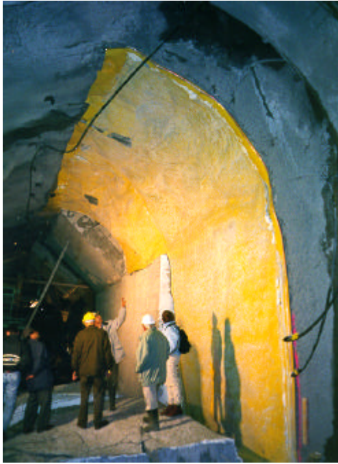
Figure 8: View of the partially exposed waterproofing membrane in the experimental gallery, the concrete support shell lies on the bottom
