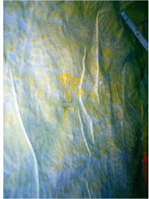
Figure 9: Vertical folds of the PVC-P waterproofing membrane, extending up to 5 cm into the concrete
