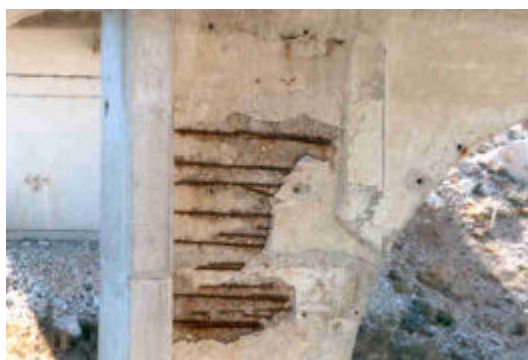
Figure 5. Krk Bridge - damage of the concrete column
