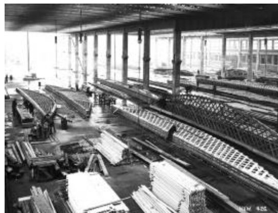
Figure 6. Fabrication of Belfast trusses c1917 (© UFTM no.426)
