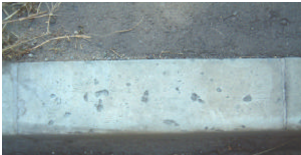
Photograph VII. Popouts on the surface of curb after 2 years (Road A, W/C: 49.5%, with waterproof agent)
