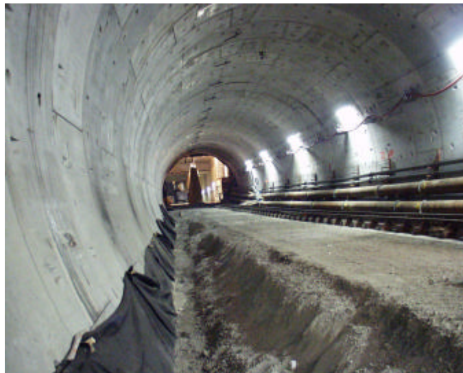
Figure 4. Lining of the Western Scheldt Tunnel with prefabricated concrete segments
