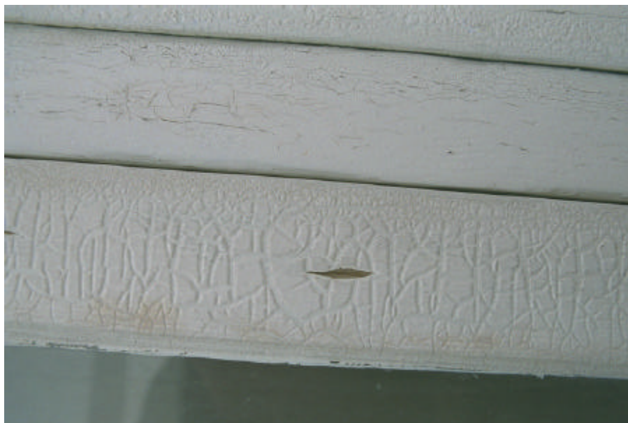
Figure 5. Paint looking like crocodile skin due to application in too thick layers.
