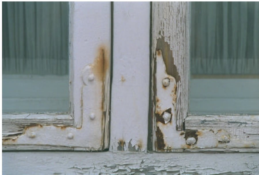
Figure 3. Bad performing linseed oil paint after about two years of exposure. Probably the problems encountered are due to insufficient cleaning of the window before application combined with poor workmanship and unfavourable weather conditions at application. The photo also demonstrates that linseed oil does not provide sufficient protection to sash-angles and other metal parts.
