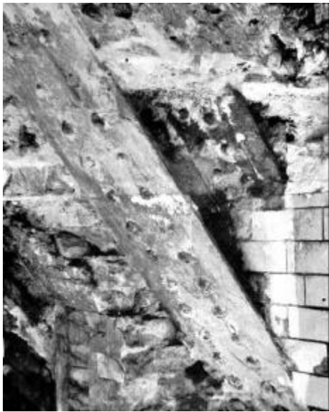
Figure 1. Early 20 th C steel frame showing corrosion, as reported in 1947.
