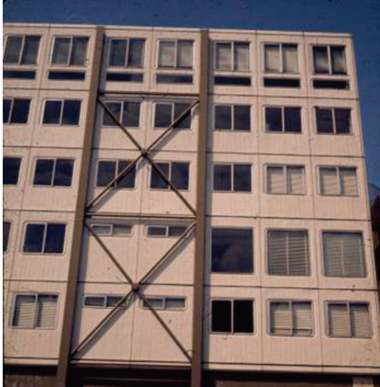
Figure 4: Five panel options produced by Jean Prouvé out of the same mould
