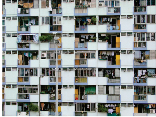
Figure 6: Old housing block in Hong Kong
