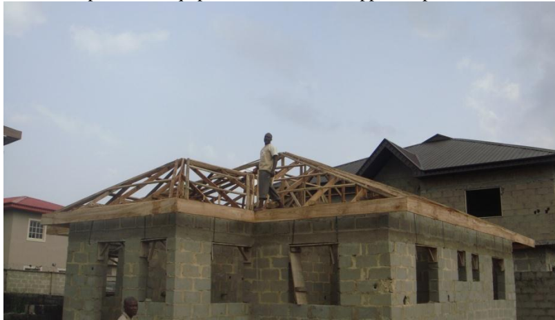
Figure 1: Worker at roof top of ongoing construction in Lagos not equipped with any safety or personal protective equipment. No scaffold support in place either
