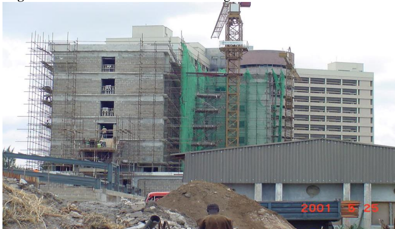
Figure 3: Another construction site in Lagos with well structured scaffold
