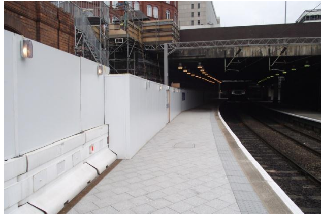
Figure 5: Platform 1 with hoardings
