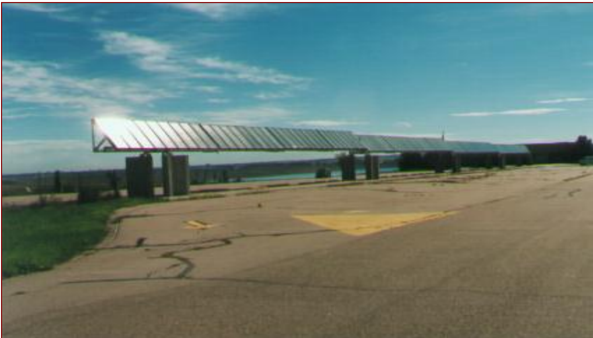
(a) solar hot water heating system abandoned in place due to mismatch with maintenance capabilities
