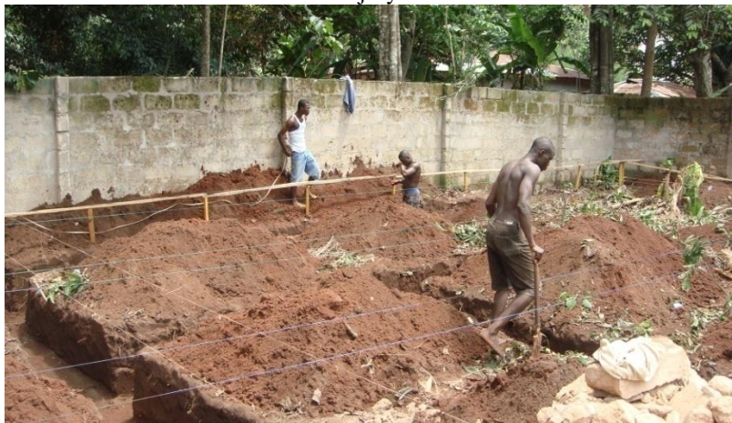
Plate 2: Site workers during preliminary construction at a site in Lagos working barefoot. Highly subject to foot injury
