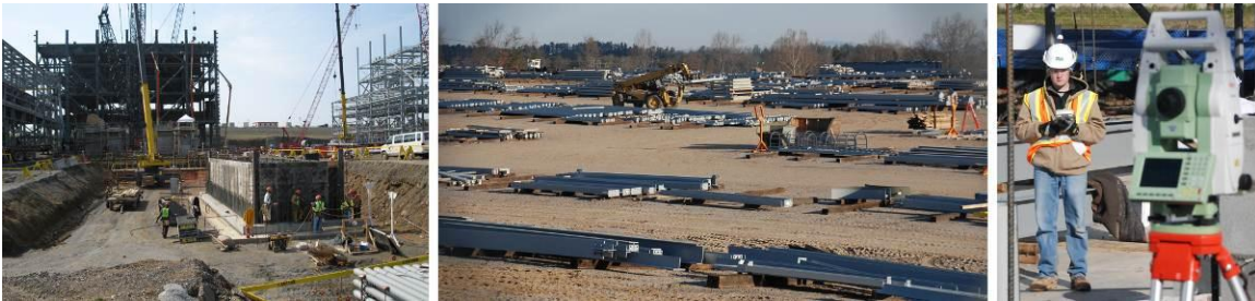
Figure 3: Layout of experiments: Construction pit (left), lay down yard (middle), and UWB tag and RTS prism on helmet (right).
