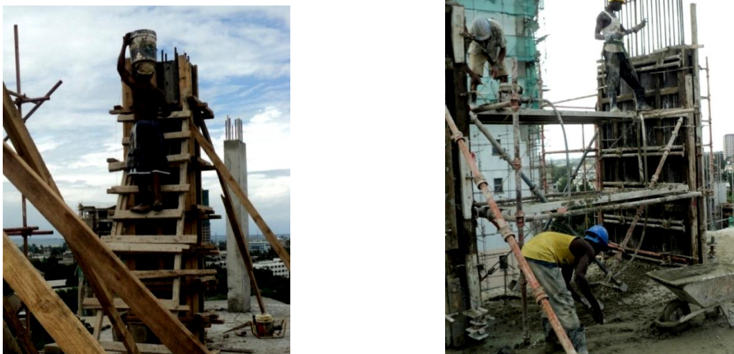
Figure 3. Concrete transportation and compacting in a construction site
