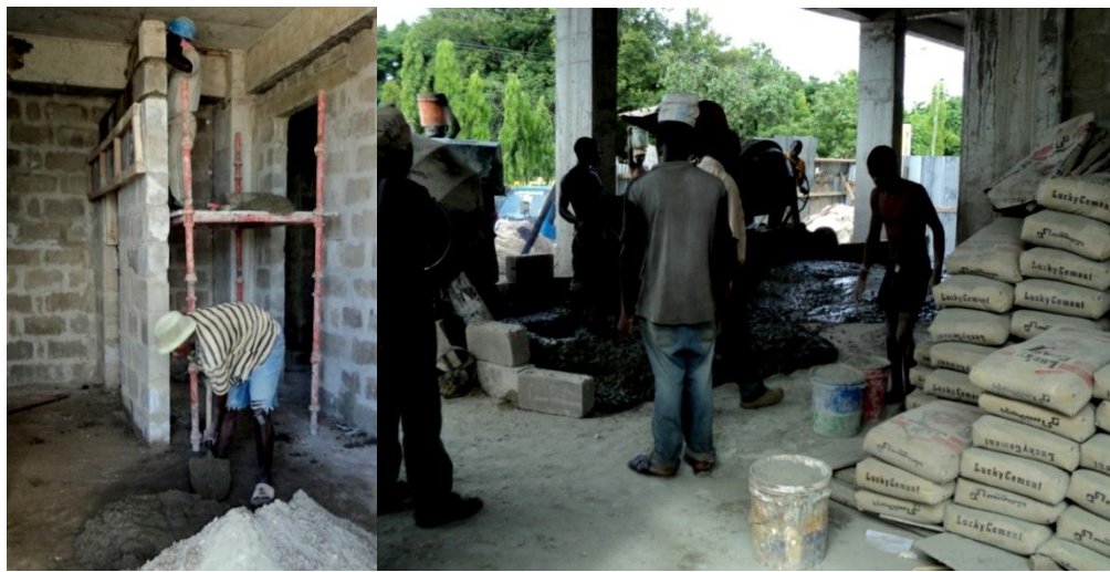
Figure 2. Block layers and a concrete casting gang at a construction site
