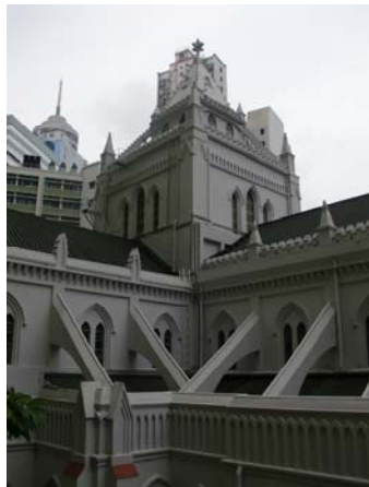
(a) Buttress structure of the Cathedral
