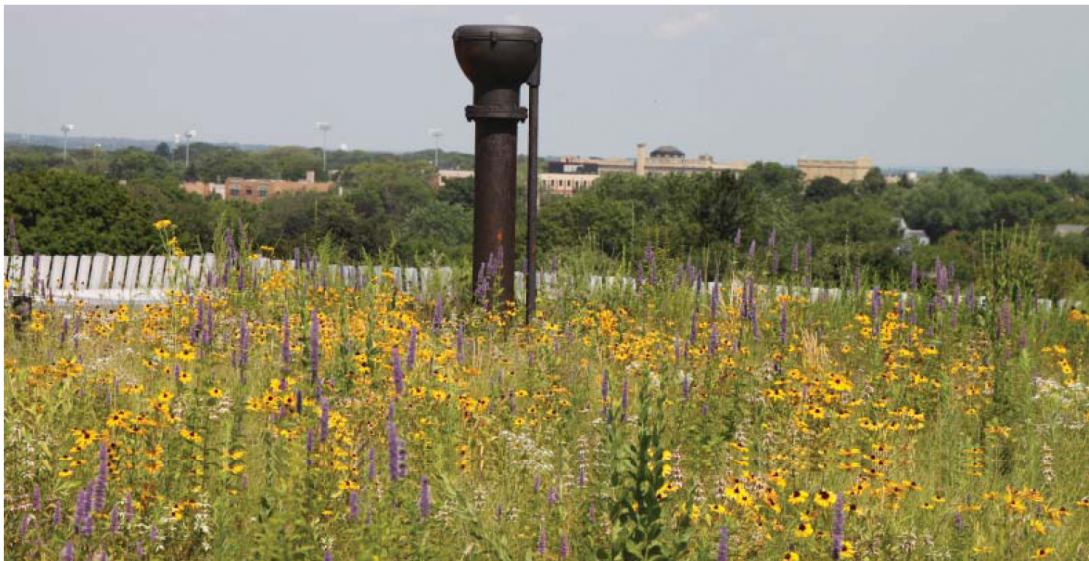
Figure 6. Sandburg Commons Green Roof. The mechanical penthouse of the commons is planted exclusively with Wisconsin native and endangered dry prairie plants, which have survived as well in four inches of substrate as the sedum of the main roof while providing habitat for butterflies and the like.
