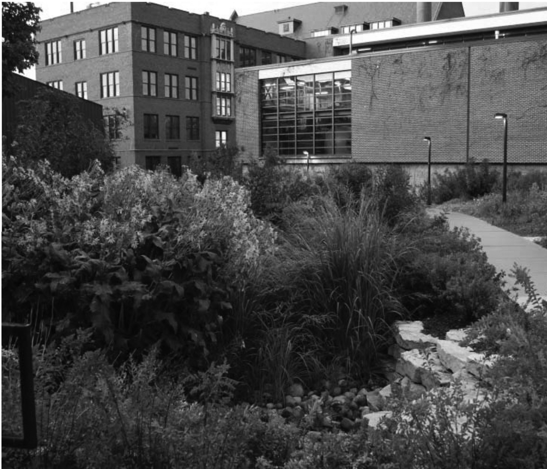
Figure 10. The Spiral Garden. This basin is the largest in a series of gardens that capture run-off from the surrounding hardscape. The Power Plant Cisterns will add both capacity and drama, bringing water through the wall of the Power Plant in the center of the second bay into Cistern 1 and ejecting overflow water from Cistern 2 at the location where the photograph is taken. Together they form the northern gates of the Pavilion Gateway Project.
