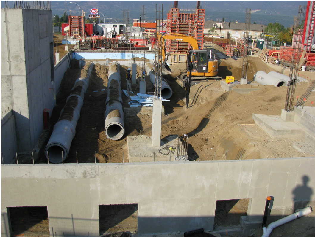
Figure 1. SASCU earth tube system under construction, 2012.
