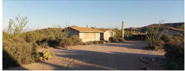
Figure 1: Existing cabins on the South East part of the site
