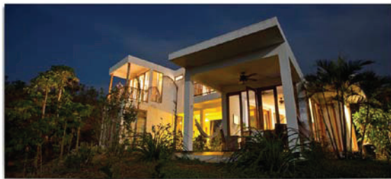
Fig. 6: South-eastern elevation, deep overhangs.
