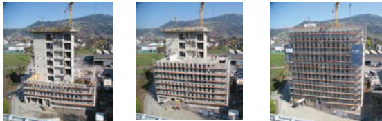
Fig 6: LCT ONE: Day 2, 4 and 8 of installation process
