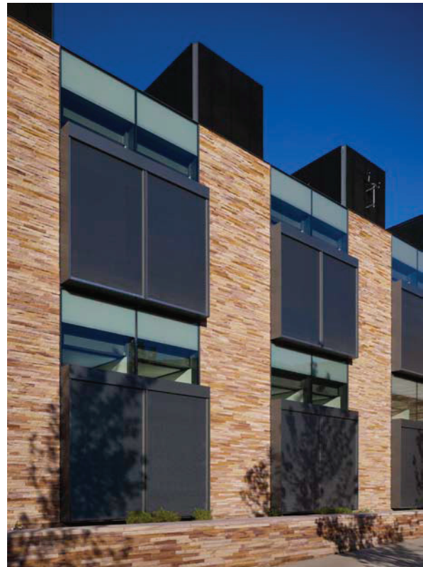
Fig 4: Automated screens at south façade in lowered position.
