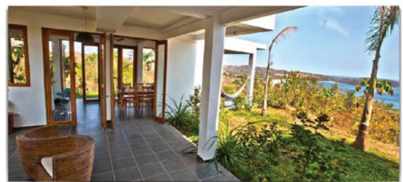
Fig. 8: Thermal mass stone slab in threshold.
