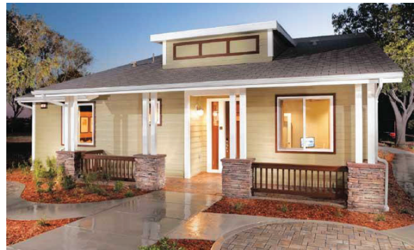
Fig. 1: ABC Green Home ZNE demonstration project
