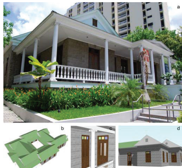
Fig. 2 Details of the González-Cuyar residence, an example of Turn-of-the-Century architecture in San Juan: a. main façade, b. wood and zinc roof detail, c. louvered doors, d. back façade.
