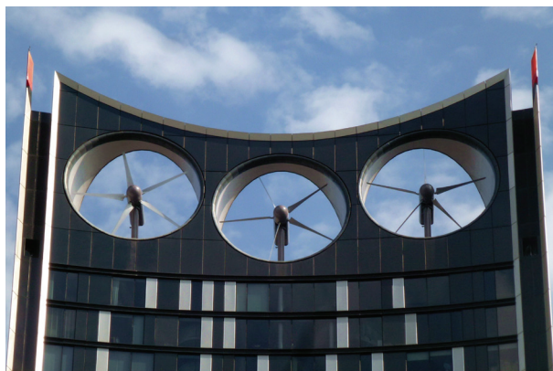
Fig.3: Wind Turbines on Strata SE1 Tower
