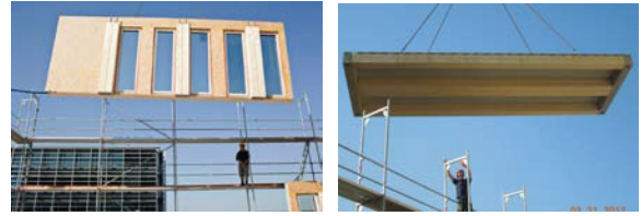
Fig.2: Prefabricated timber wall & floor panels for LCT ONE
