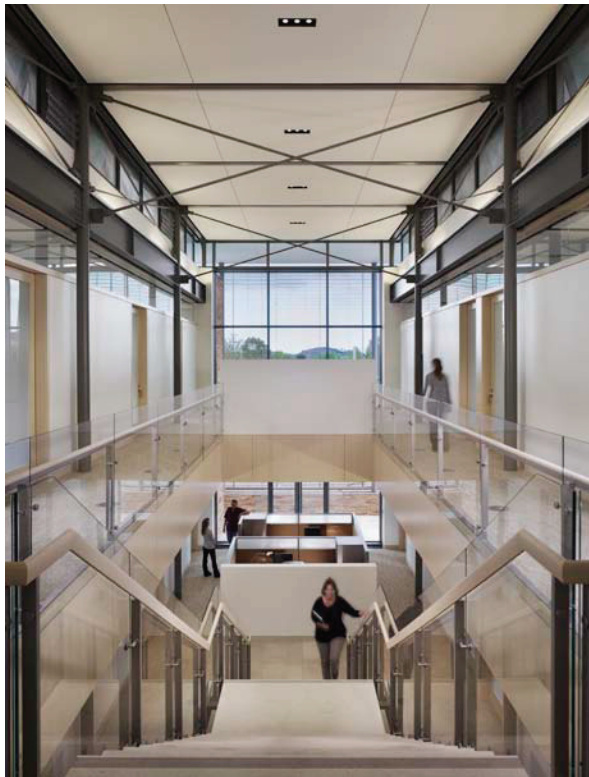
Fig 5: Air is expelled through digitally controlled clerestory windows at top of atrium.
