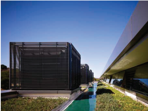
Fig 3: Passive downdraft chimneys at rooftop.
