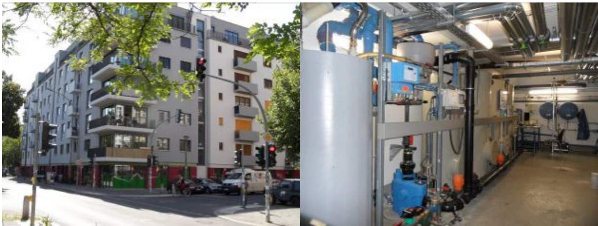
Photo 1: Greywater recycling combined with heat recovery in a multi-storey passive house in Berlin, Germany (Photos: E. Nolde).
