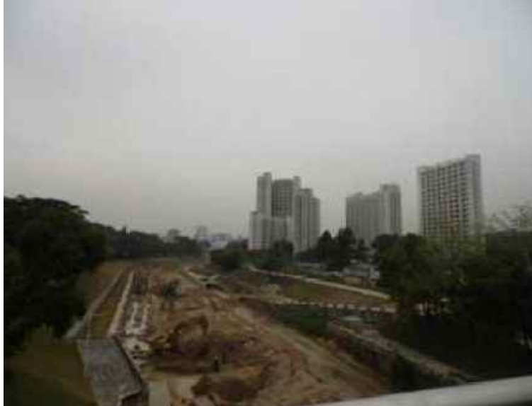
Figure 4: In the beginning of construction of a building site in Shenzhen.
