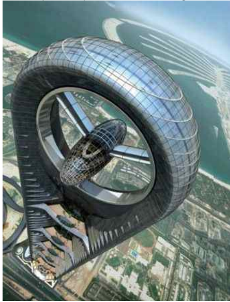
Figure 1: Anara Tower (Picture by Atkins Design Studio).
