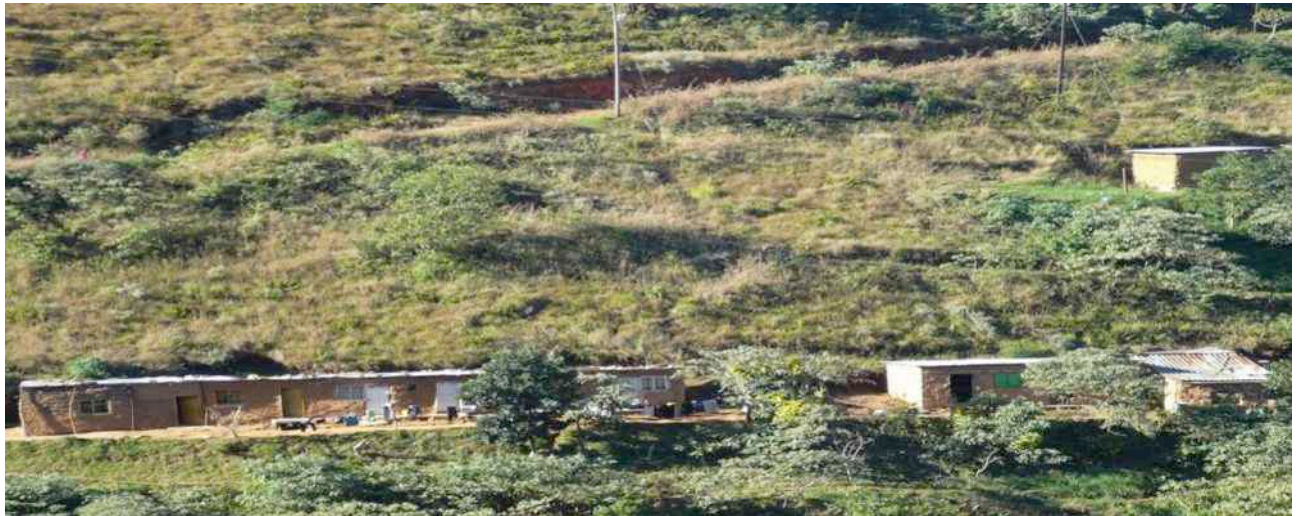
Figure 1 Informal settlement before the construction of trunk infrastructure, services, and improvement of major roads (Cities Alliance 2014).
