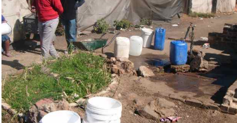
Figure 5: Greywater Management through vegetated soakpit in Makause Settlement, Ekurhuleni (Author’s Photograph, June 2013).
