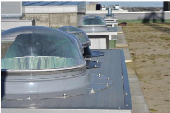
Fig 3 - Tubular daylighting devices (Solatubes) in green roof
