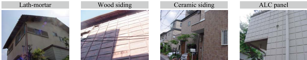
Fig. 3 Exterior wall photographs
