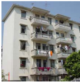
Fig. 1 Original Southern Façade
