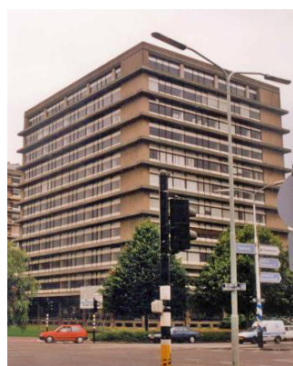
Figure 2: The building depth of the existing building provided open, spacious floor plans. 2 of the 4 elevators were not needed and were reused for shafts or included in the apartments.
