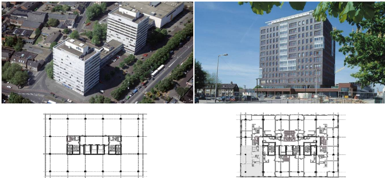
Figure 2: Twentec building. Left the building before conversion, to the right the building after conversion.
