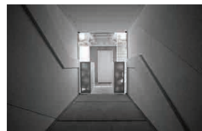
Fig. 8 New Floor Installed in Vacant Stairwell
