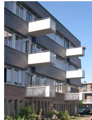
Figure 1: The 5,4m structural grid enhanced the conversion capacity. The existing facade was upgraded by placing new windows, insulation and balconies. An additional floor was added on top of the building.
