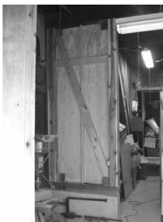
Photo 12. New Structural Element on Earthen Floor (K1)
