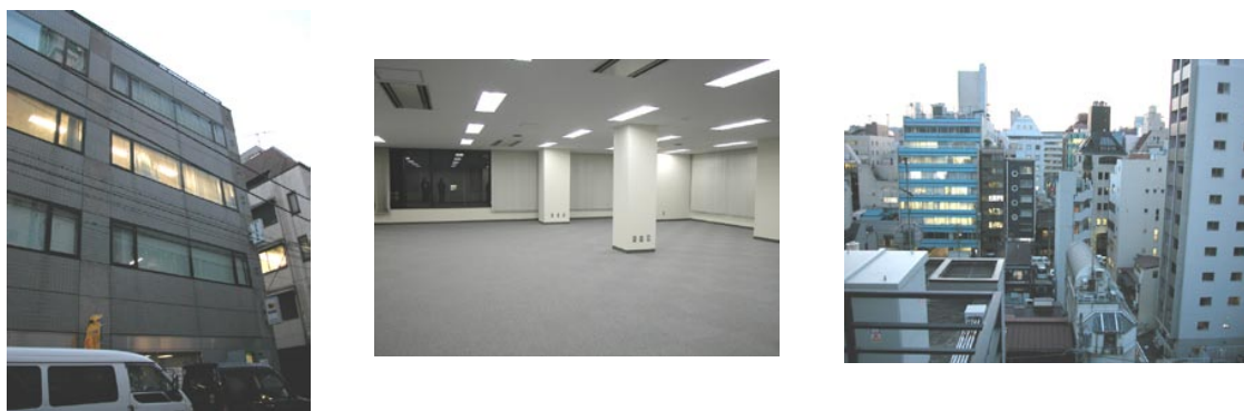
Fig. 1 Y Building before Conversion and its Surroundings
