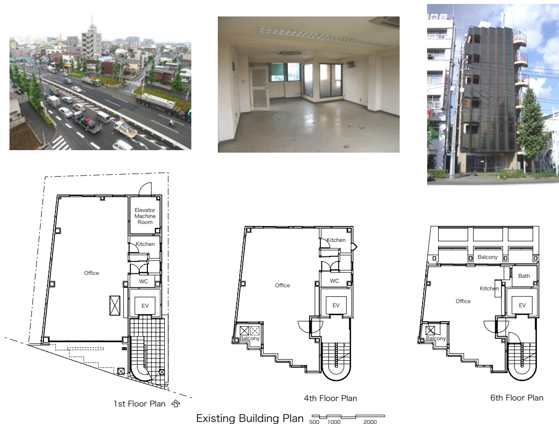
Fig. 5 G Building before Conversion and its Surroundings
