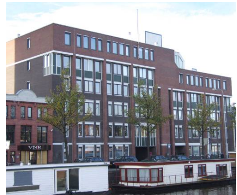
Figure 3: The building had operable windows in every bay and was converted from office building to student housing without altering the facade. The floor lay-out with a central elevator caused an awkward routing.
