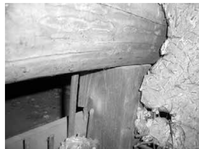
Photo 3. Column-Beam Connection (K2)
