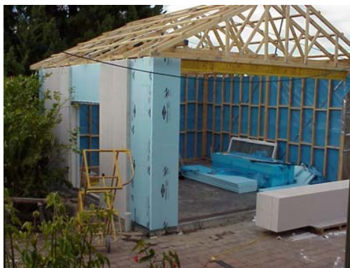
Figure No 3. Supatherm system applied to a timber structural frame
