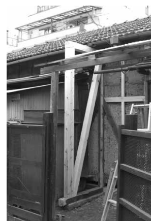
Photo 6. Reinforcement by Wooden Brace (No.7)
