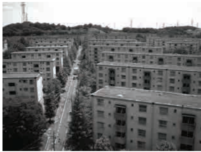
Fig. 1 Housing Estate Built in the Mass-housing Era
