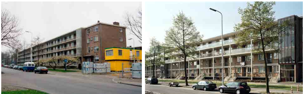
Fig. 2 Enschedlaan, The Hague (before and after rehabilitation)
