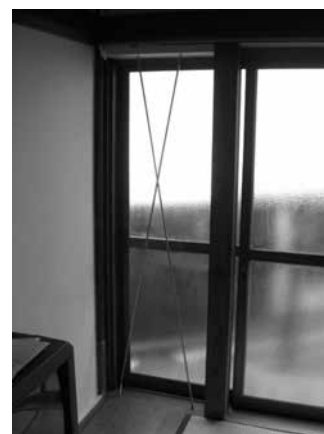
Photo 13. Reinforcement by Stainless Steel Brace on Openings (K2)
