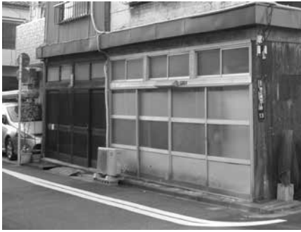
Photo 7. The Openings in the Ridge Direction (N)
