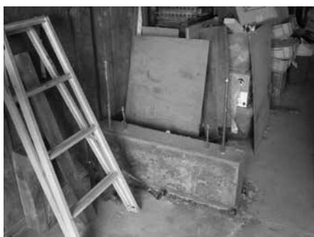
Photo 11. New Foundation on Earthen Floor (K1)
