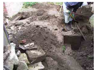
fig.13 Duct of the Chimney and Remains of the Fire Place
