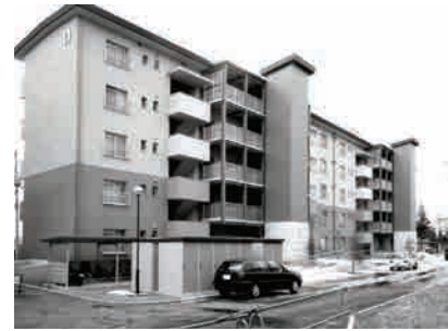
Fig. 3 Residential Building with Added Access Corridors
