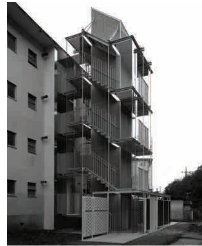
Fig. 6 Experimental Elevator Addition System
