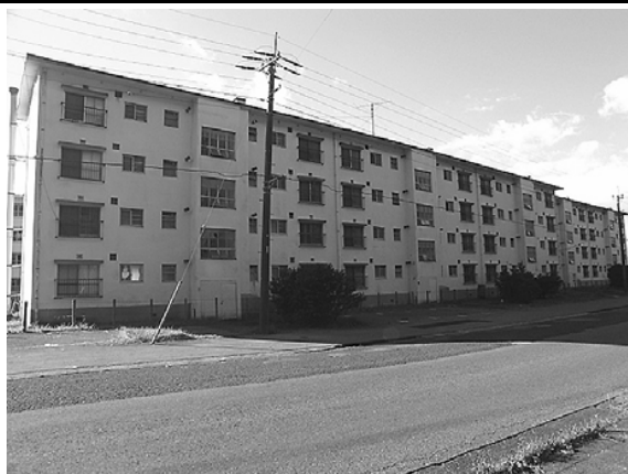
Fig. 1 Building before renovation
