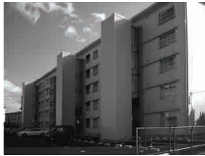
Fig. 2 Residential Building with Added Elevator Towers
