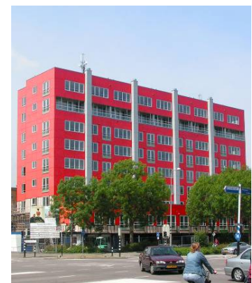
Figure 4: The prefab curtain wall could not be altered and was replaced. The cantilevering of the floors made it impossible to add balconies.
