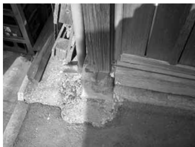
Photo 2. Column Base (K1)
