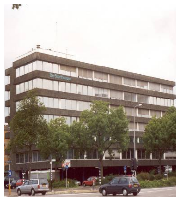
Figure 4: The prefab curtain wall could not be altered and was replaced. The cantilevering of the floors made it impossible to add balconies.
