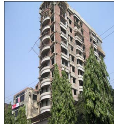
Fig. 7 High-Rise Construction by Formal Private Developer
