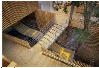
Photo 6: The floorboard was made of hinoki (25mm × 110mm), The outside and inside wall was made of cedar(25mm × 180mm)
