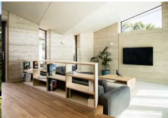
Figure 3 Rammed earth walls at Passive Butterfly. Photography by Amorfo.
