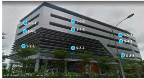
Figure 2 Location and alignment of measuring points at the affected building.
