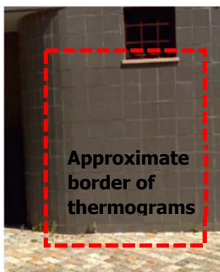
Picture of an adhered ceramic cladding with delamination
