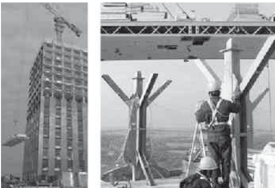
Fig. 1: On-Site Assembly and Installation Processes at T30A Tower Hotel, BSB Sustainable Building
