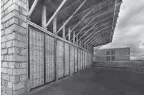
Workshop building constructed by a group of student during a design-build project near Nairobi, Kenya
