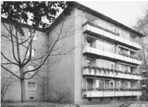
Fig. 1: Balcony facade before the refurbishment [1]
