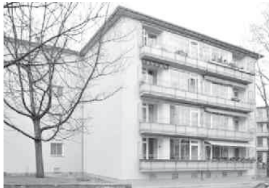
Fig. 2: Balcony facade after the refurbishment [1]
