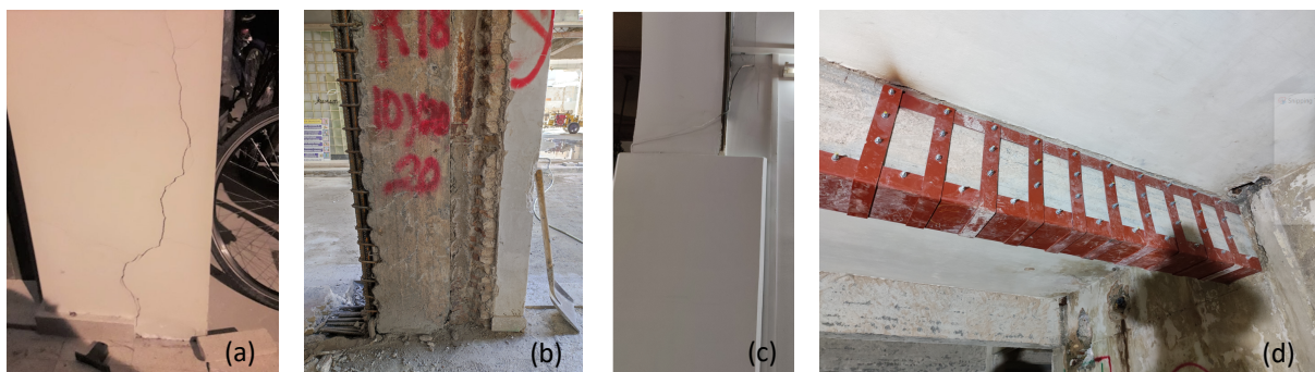
Figure 1: (a) Crack expansion in restored column due to expansion of corroded steel reinforcement, (b) Strengthening of column only on one side, (c) jacketing of column only up to a certain height, (d) externally bonded reinforcement of beam
