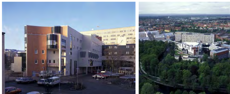
Figure 4. Exterior and aerial view of the O-building
