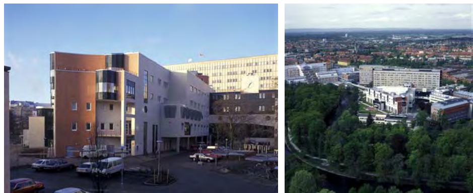
Figure 4. Exterior and aerial view of the O-building
