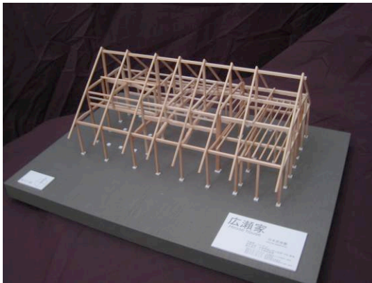
Figure 4 Framework model of the Hirose Residence
