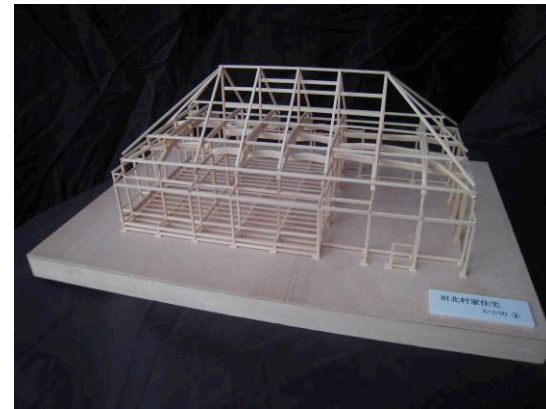
Figure 5 Framework model of the Kitamura Residence
