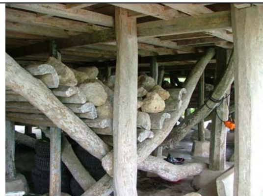
Detail of bracing and weighting used for increased friction & earthquake resistance
