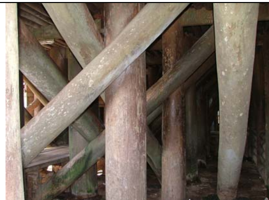
Bracing and piles below the Chiefs house
