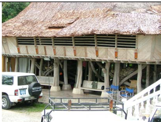
A traditional house in Gunung Sitoli with bracing and piles on stone blocks
