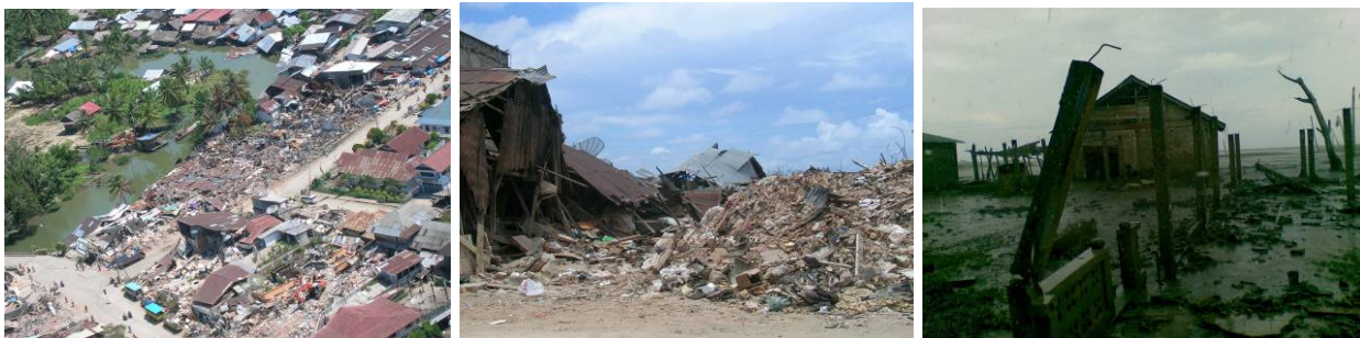
Destruction by earthquake in the town centre of Gunungsioli (Photos: Unknown 2005), and by Tsunami in Idanogawo (Photo H.Lang, 2008).
