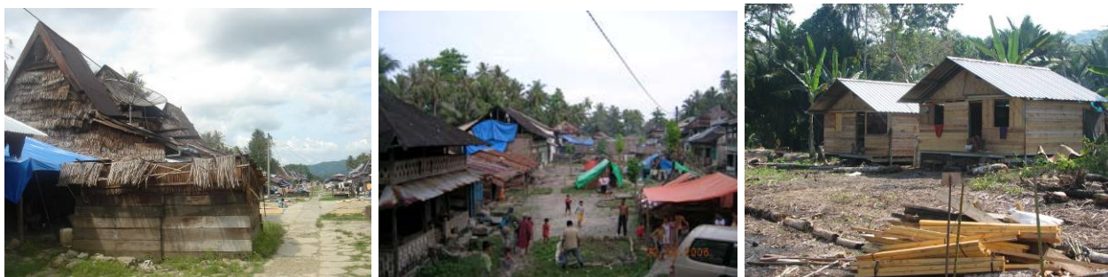
Temporary shelter built by the survivors in Bawogozali village, South Nias (Photos H.Lang 2006), and transitional shelter financed by IFRC (Photo B.I. Wibisono, 2007)
