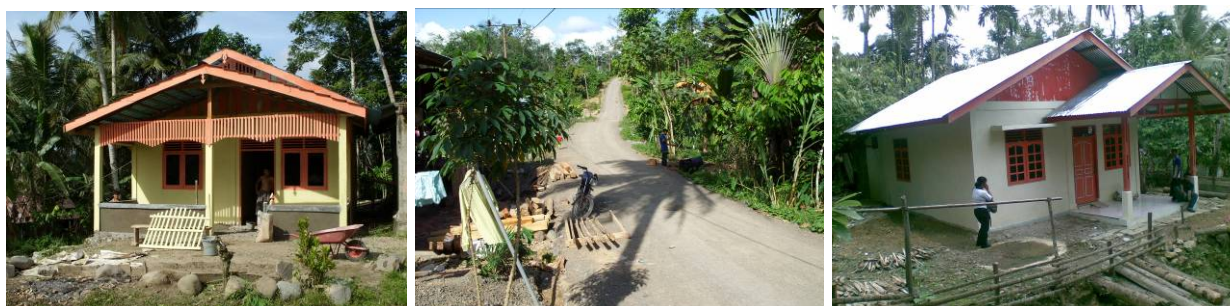
A finished house in Lolowau, road after construction in Lolowau (Photos B.I. Wibisono 2007), and a house in Situlu Ori (Photo H.Lang 2008)
