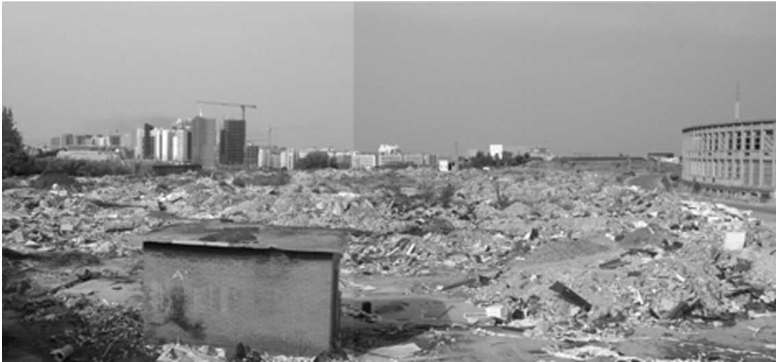
Figure 1. Illegal Construction and demolition dump in abandoned factory in Lisbon
