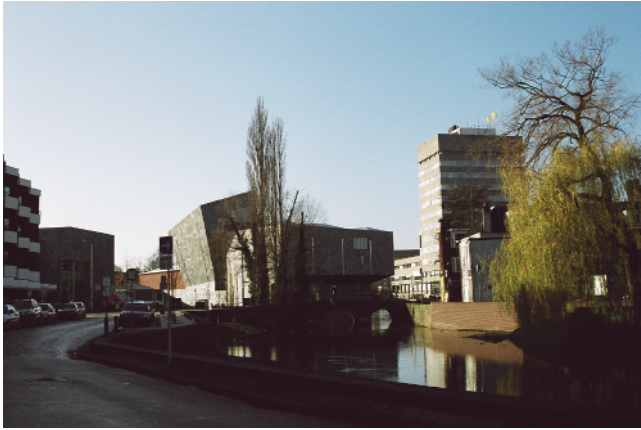
Photograph 3. The back side view of Van Abbemuseum through new wings (photo by Y.K.Aktuglu, 12/2006) .
