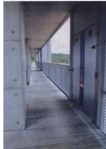
(2) Pipe shaft installed in the common section
