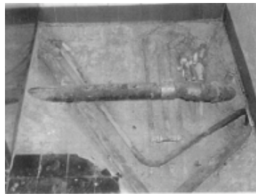
Figure 9: Pipes set in concrete
