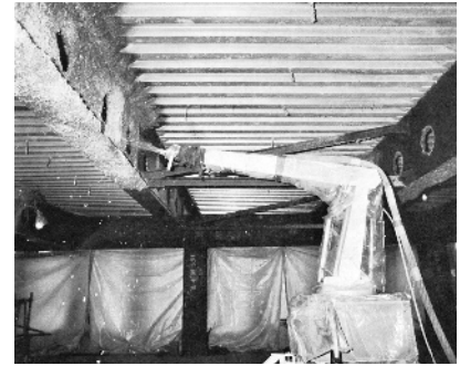
Fig.2 Fireproofing Spray by SSR-1
