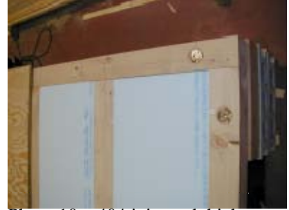
Photo 10 404 joist and thick plywood floor sheathing.
