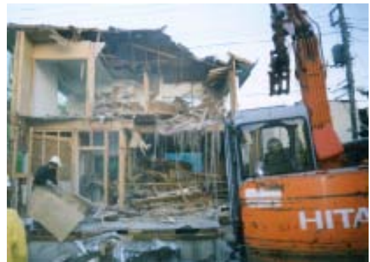
Photo 2 Wood frames demolished by machine.
