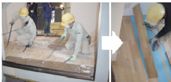
Photo 12 Hard wood floorings removed. Right: "Improved". Flooring can be easily removed without damaging the floor sheathings and floorings.
