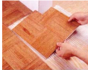
Figure 1. Installation of the flooring (Current design) – Floorings are nailed and glued to the floor sheathing.
