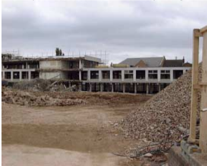
Figure 4. Demolition of structures following soft strip
