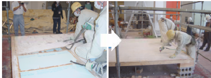
Photo 15 Floor sheathing removed. Right: “Improved”. Floor sheathings can be easily removed when they are not glued to the floor joists and connected by wood screw.
