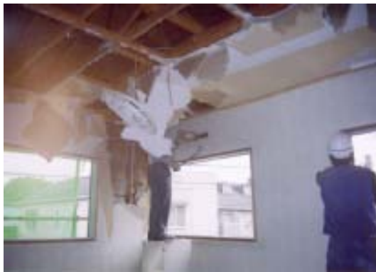
Photo 1 Gypsum boards remove by hand.
