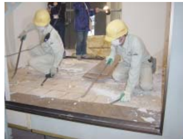
Figure 2. Removal of the flooring (Current design) – Floorings are removed by using deconstruction tools. Wood pieces and adhesive remains on the floor sheathings.
