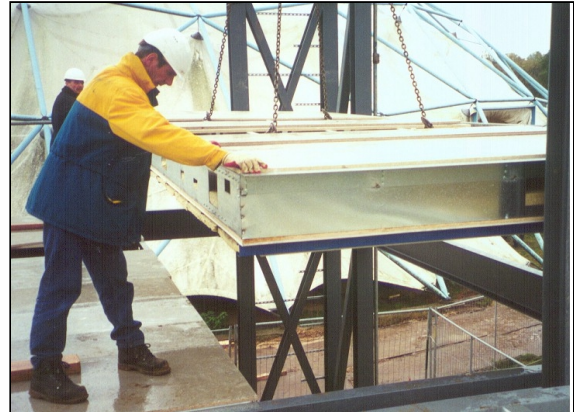
Figure 2. Assembling the floor panels.
