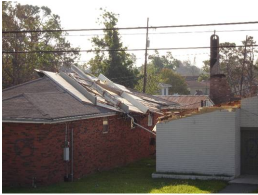
Figure 7. Removal of a church roof from the supporting walls.
