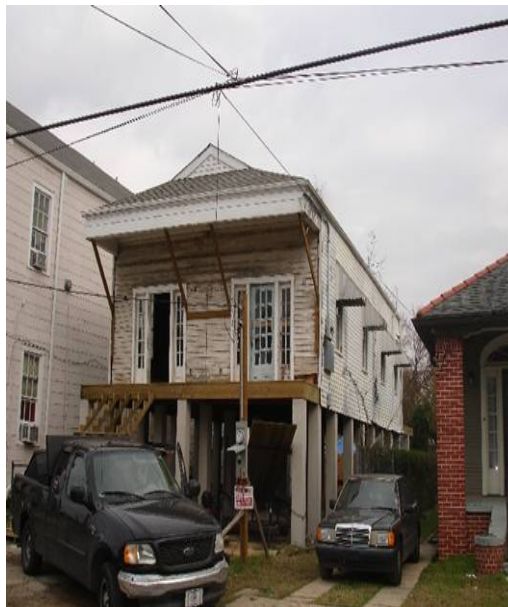
Figure 6. Structure recently elevated to above the BFE.
