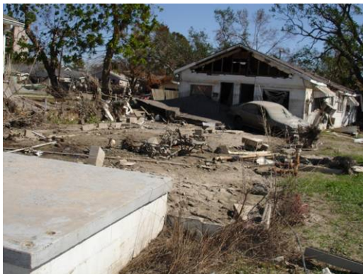
Figure 1. One story timber frame structure pushed away from the concrete porch.
