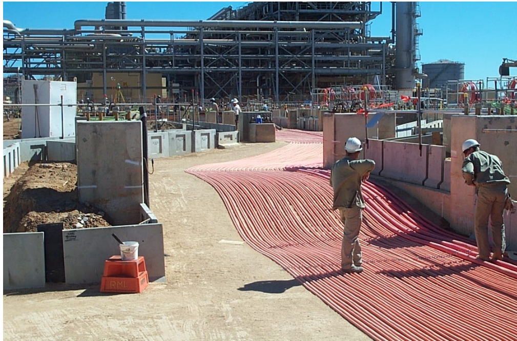
Plate 5.1 –Site Housekeeping – Woodside LNG Train 4
