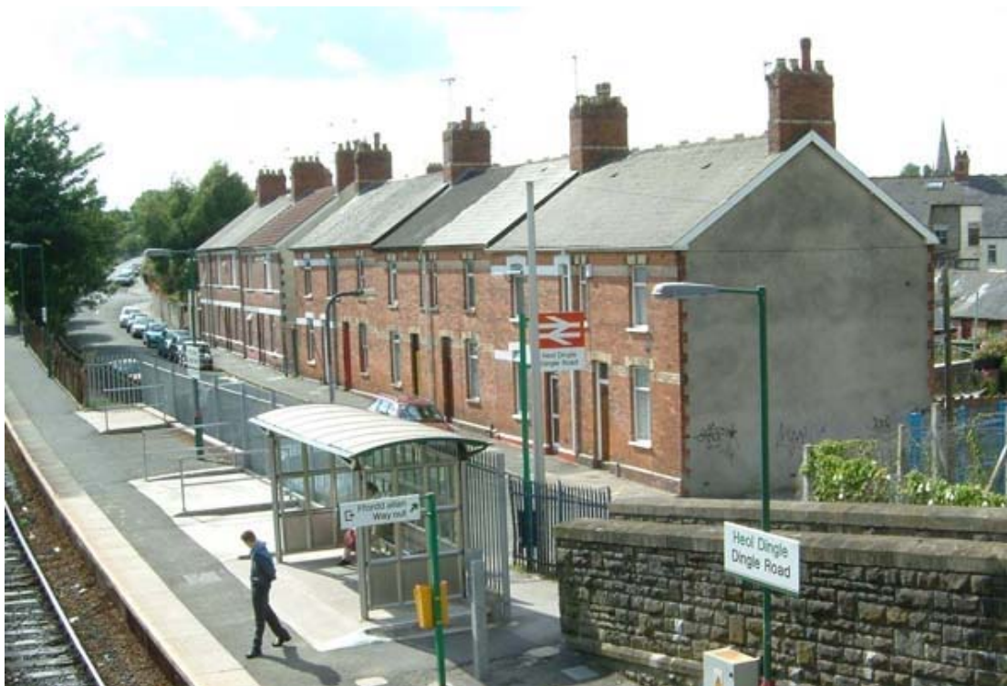
Dingle Road station after improvements
