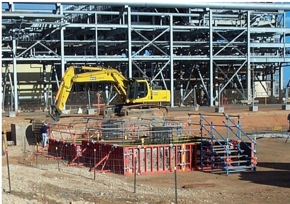
Plate 5.2 –Foundation Construction Access and Barriers Woodside LNG Train 4
