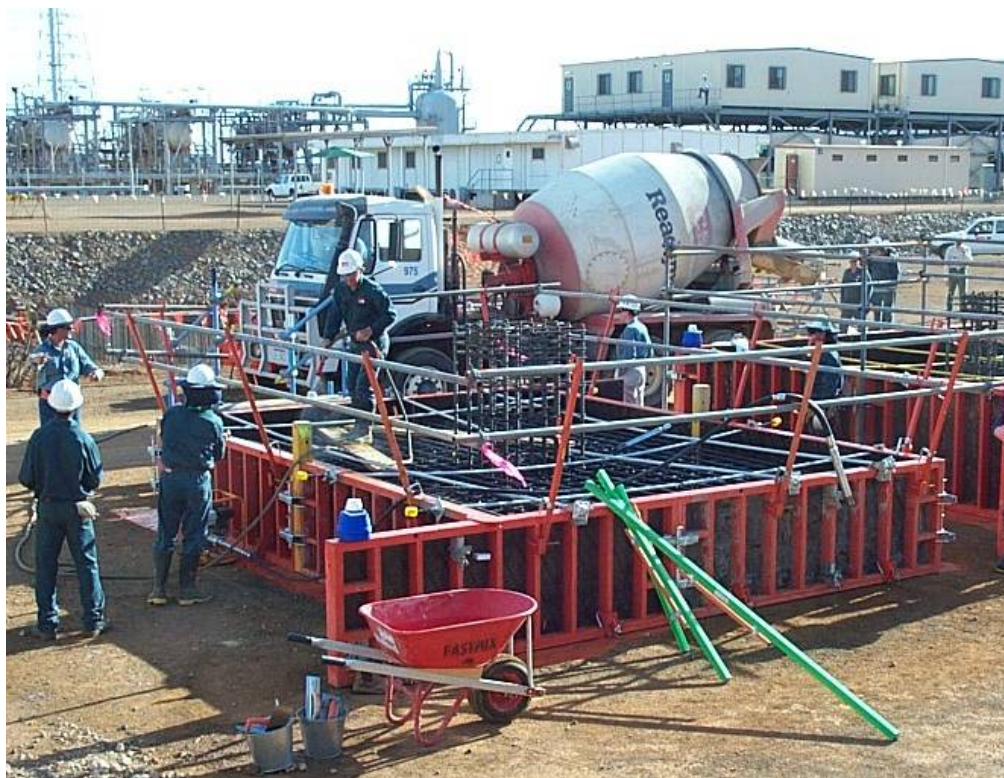
Plate 5.3 – Foundation Construction Access and Barriers - Woodside LNG Train 4
