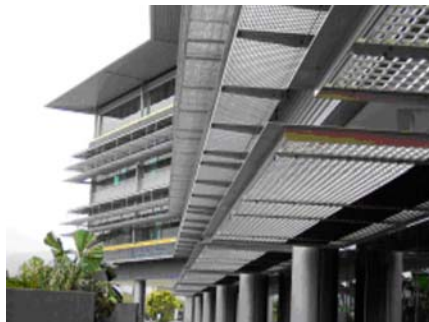
Figure 4 Shades For Maintenance
