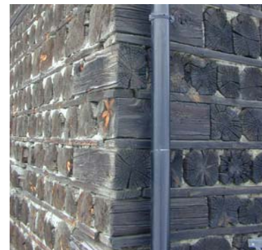
Figure 12 Vernacular “Log masonry” used in a barn from 1840 at Ner-Skjørstad in Oppdal, Norway. [3]
