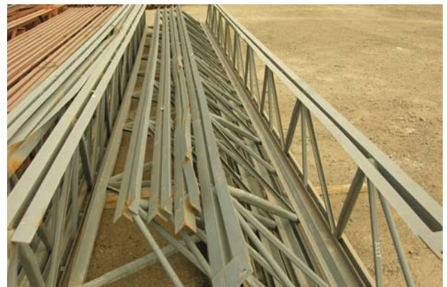
Figure 3: Open web steel joists can often be dismantled for reuse, but the new structure needs to be designed around the available spans.
