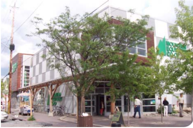
Figure 1: The Mountain Equipment Coop has pioneered component reuse in many of its retail stores. This one located in Ottawa reused many parts of the previous building on site, including the foundations.
