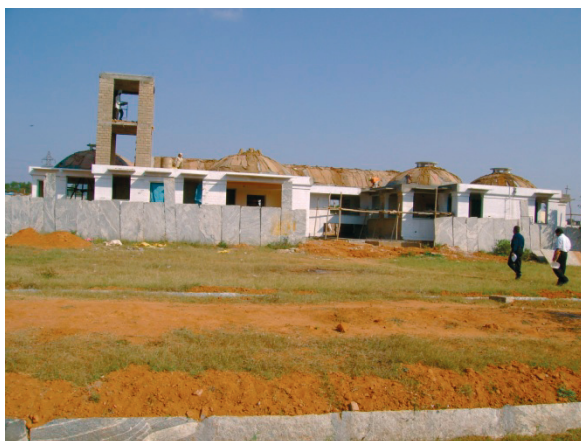
Figure 4 Large house with vaults and domes
