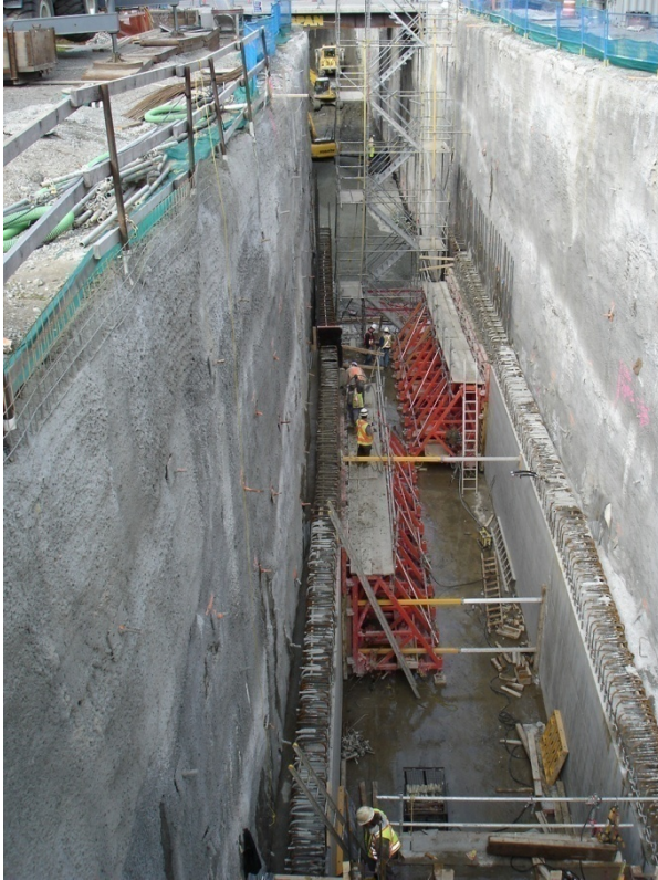
Figure 5. Stacked cut and cover tunnel
