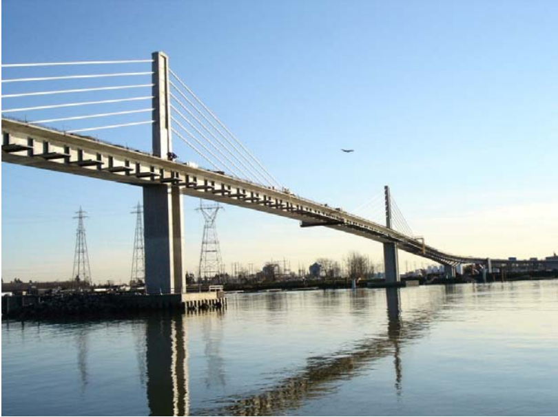
Figure 3. North Arm Bridge
