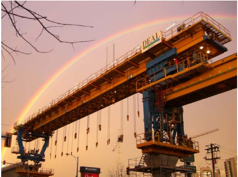
Figure 2. Segment erection truss
