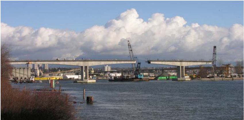
Figure 4. Middle Arm Bridge
