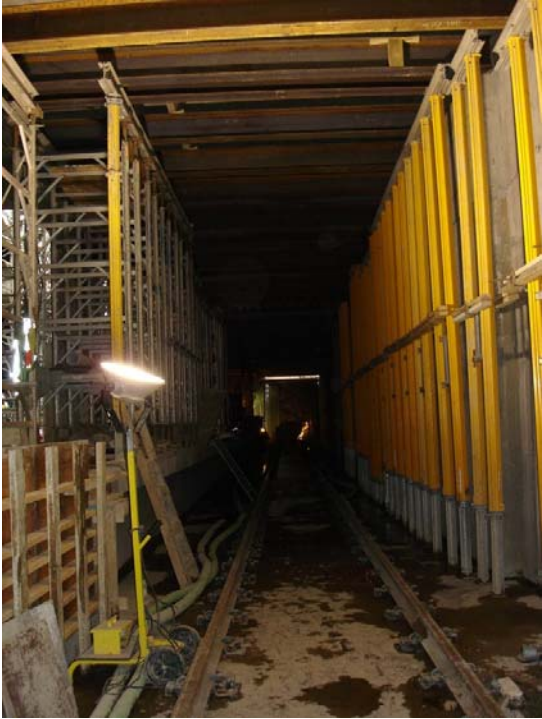
Figure 10. Shoring above tracks
