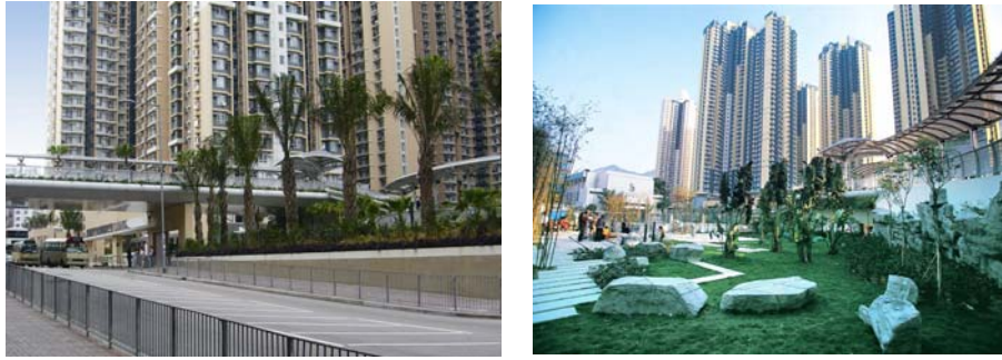
Figure 4: The footbridges connecting Phase 4 and Phase 5; and the Bamboo Garden in Kwai Chung Estate Phase 5 with Phases 3 and 4 beyond
