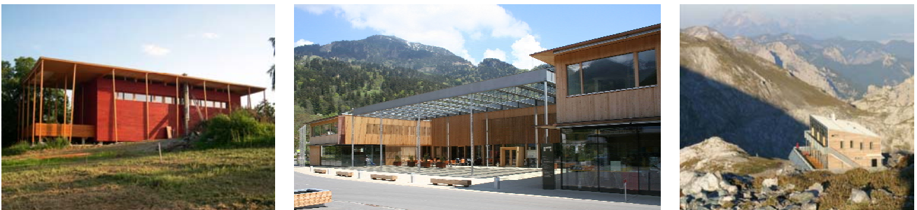
Figure 4: Special buildings in passive house standard. From left to right: S-house (Wimmer, 2005) (Source: GrAt, Schleicher Architects), Gemeindezentrum Ludesch (Source: Gebhard Bertsch, Hermann Kaufmann Architects), Schiestl House alpine refuge at Hochschwab 2154 m above sea level (Source: Treberspurg & Partner Architects, pos Architects)
