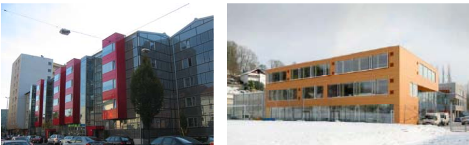
Figure 5: Buildings with thermal retrofit measures that meet the passive house standard. Left: Housing estate Makartstrasse-Linz (Source: Robert Freund, Arch+More Architects), Right: School Schwanenstadt (Source: PAUAT Architects)
