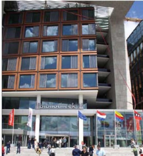
Figure 5 Photo of the newly erected Ecobuilding Amsterdam Library.
