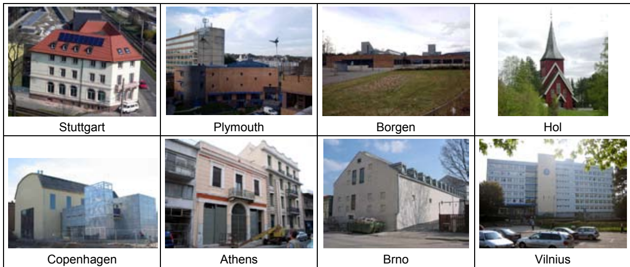
Figure 7 The demonstration buildings in the BRITA in PuBs project after the retrofits.
