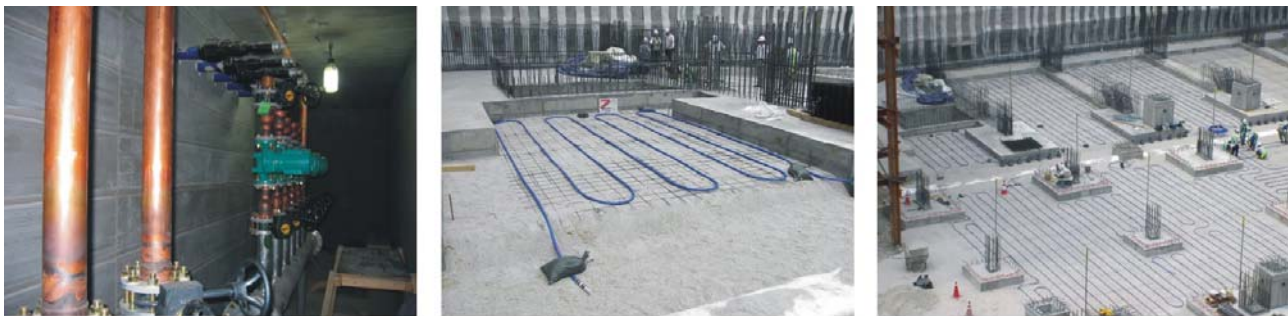
Figure 7 Construction pictures of geo-thermal buried pipes and supply header (B6F)
