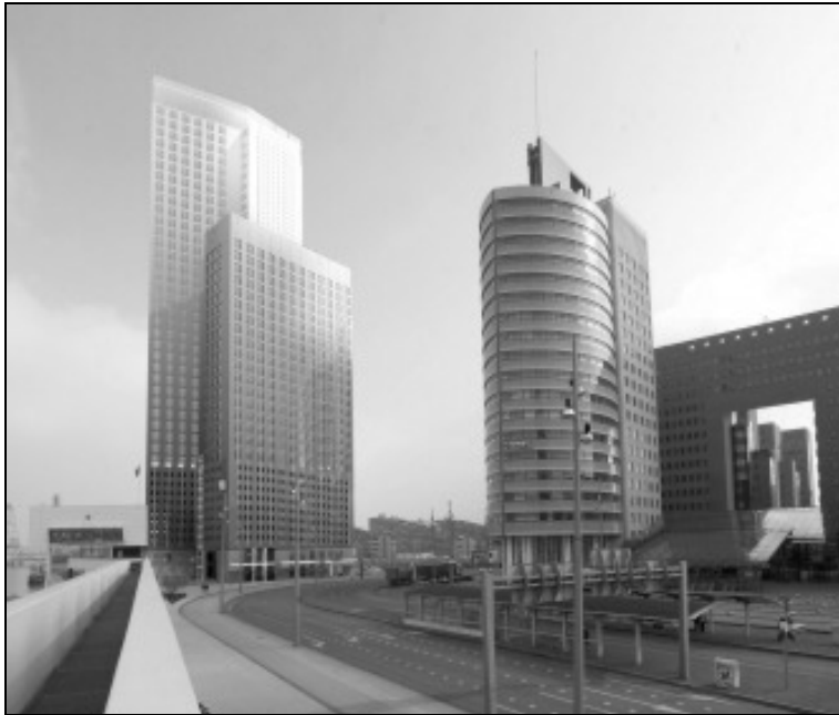
Fig. 4. Maas Tower, initiative of OVG, used for testing
