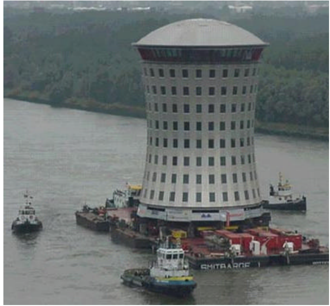
Figure 4: Construction and transport of The Bollard office building (pictures by courtesy of Mammoet and Grootint/Heerema)
