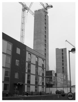
Figure 2 Modular building stabilised by a concrete core (courtesy Caledonian Building Systems)
