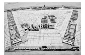
Figure 2: A Lustron house "kit" spread out on an airport runway to demonstrate the extensive contents of a Lustron House kit of parts. (ca 1950)
