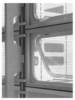
fig.19: inside view of panel fixing cramps.
