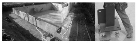
Figure 3. Left, underground floor with geothermal installation and energy supply and IT connections. Right, steel columns anchored to the foundation slab with bolted (demountable) base plates.
