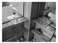
Figure 5: Bolted connections of 8 Sekisui Heim 3D modules
