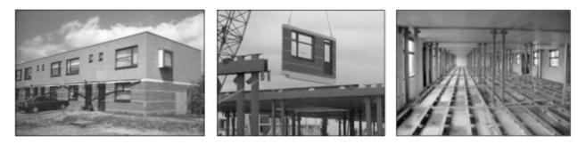
Figure 10: The objective of the IFD project A+ dwellings was to create homes that are adaptable to the composition of families and to changing housing needs. The Infra+ floor contributed to this flexibility
