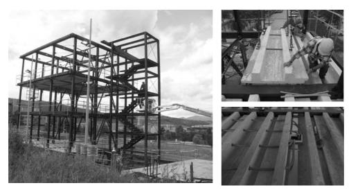
Figure 4. Demountable, floor by floor, steel structure and precast concrete slab. The steel beams and precast slabs allow building services integration.
