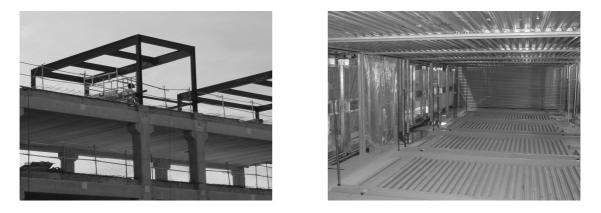
Figure 12: Manubuild Corus steel module penthouse & semiautomatic car parking
