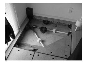
Figure 9: Next Infill raised floor with piping
