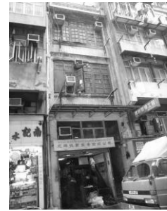
Photo (Field survey)
