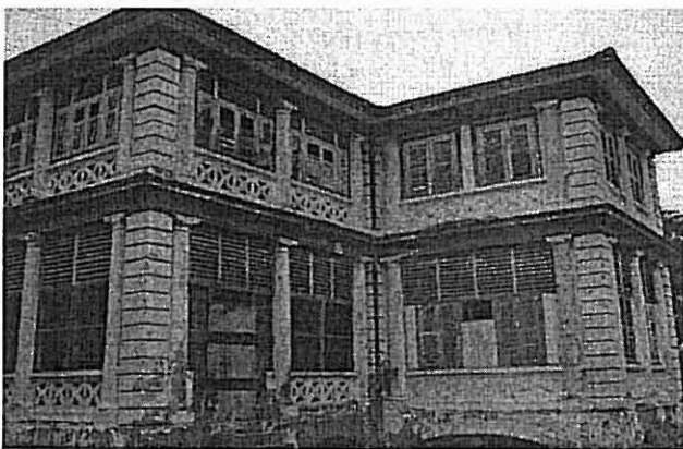
Figure 1: Case study – Before restoration (Source: www.hbp.usm.my/conservation/biodata.htm )
