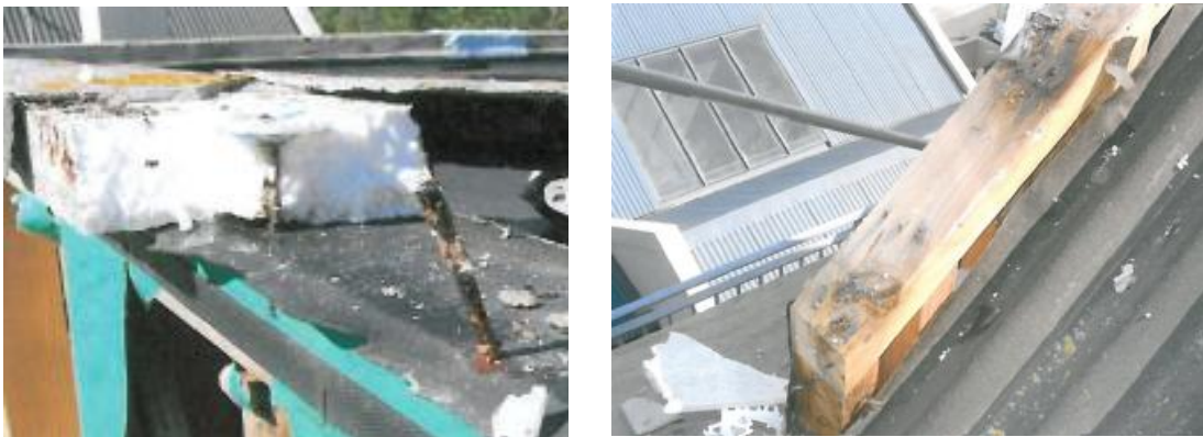
Figure 1: Examples of decay at head of parapet walls – notice lichen growth on left-hand photo
