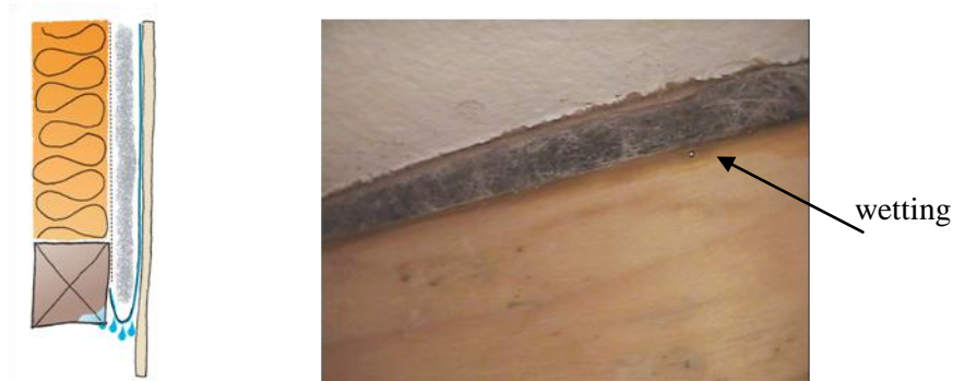
Figure 6. Frame wetting – water tracked along from bug screen
