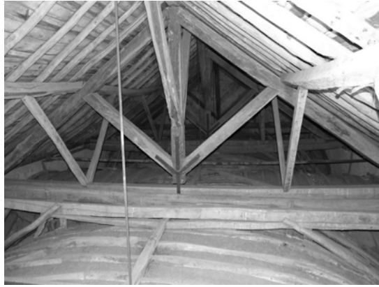
Figure 3: Loft of the covering of the central nave (XV century). Distortion of the base of the shear
