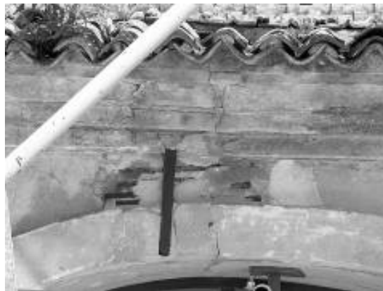
Figure 6: External envelope of the central nave.
