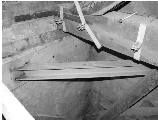
Figure 3: Loft of the covering of the central nave (XV century). Distortion of the base of the shear
