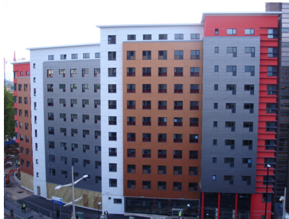
Figure 4: 12 storey modular student residence at Bond Street, Bristol (courtesy Unite Modular Solutions)
