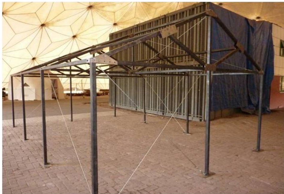
Figure 3: Pakistan steel frame for winterized shelter
