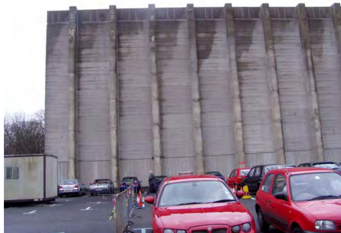
Figure 11: Obstruction Opposite Window
