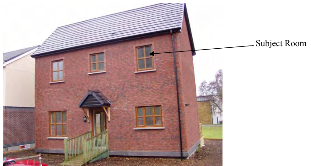
Figure 10: Outside of the Building being tested
