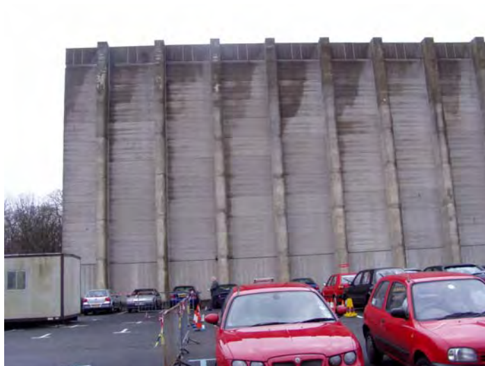
Figure 11: Obstruction Opposite Window
