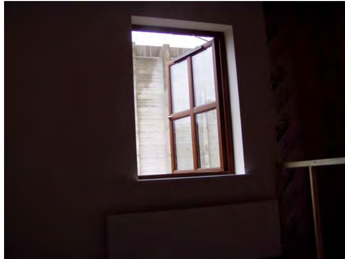
Figure 12: View from Within Room
